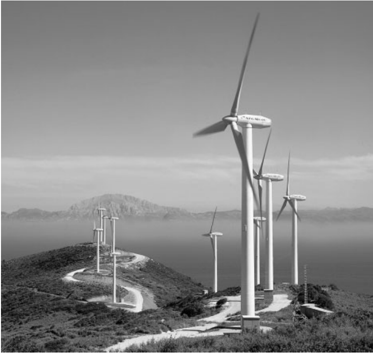
Figure 9.4 Windfarm of 600 kW, 43 m diameter Wind Turbines, Tarifa, Spain (Reproduced by permission of NEG MICON; www.neg-micon.dk )
