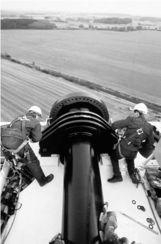
Figure 6.19 Turbine Assembly in the Air (2). (View of low-speed shaft and front bearing after installation on 1.5 MW NEG Micon turbine). (Reproduced by permission of NEG Micon)
